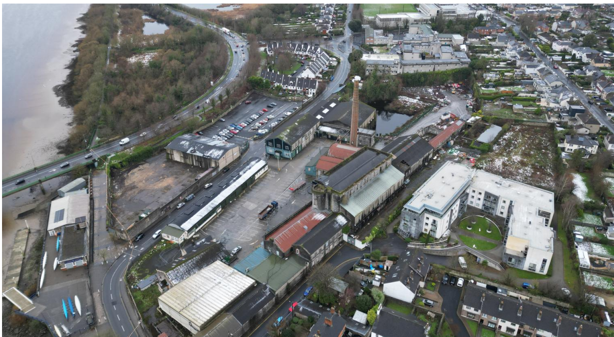
Figure 44 – aerial view of the site from the east.
