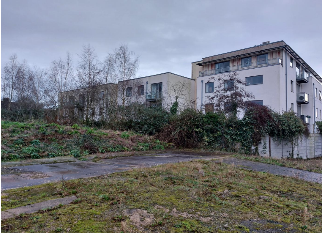
Figure 38 – View of the Stonetown Terrace plot from the upper reservoir.
