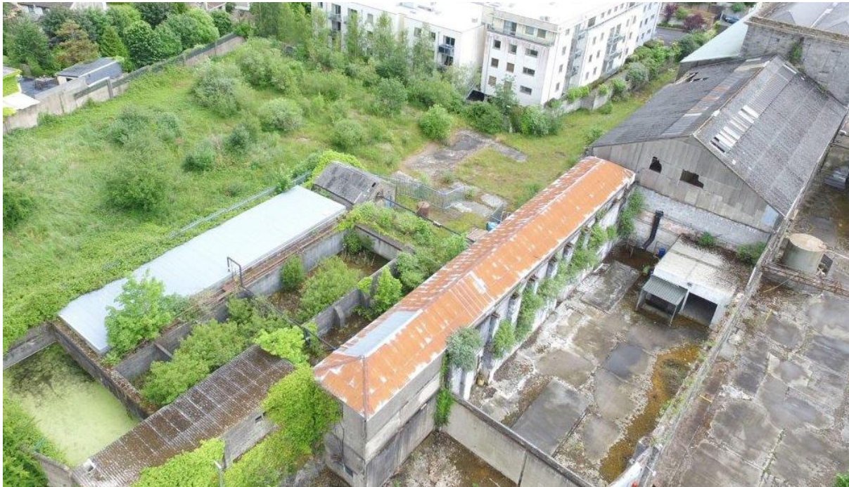
Figure 16 - Aerial view showing the long lean-to at the rear of the derelict cold store below the upper reservoir.
