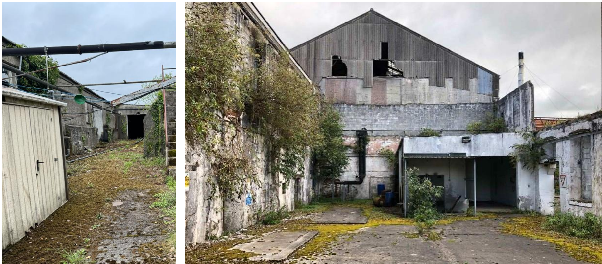
Figure 13 – North, upper aspect of the lean-to addressing the Stonetown Terrace site and a view from within.
