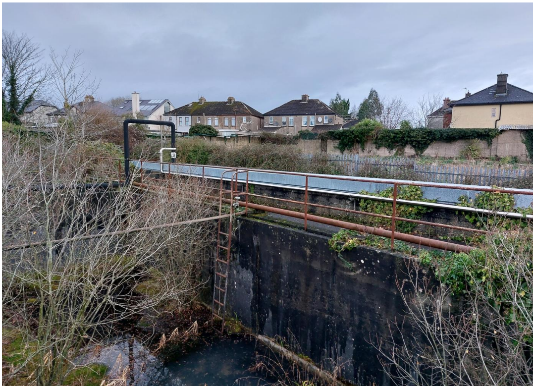
Figure 39 – looking across the tanks of the upper reservoir toward the rear of Clanmaurice Avenue.
