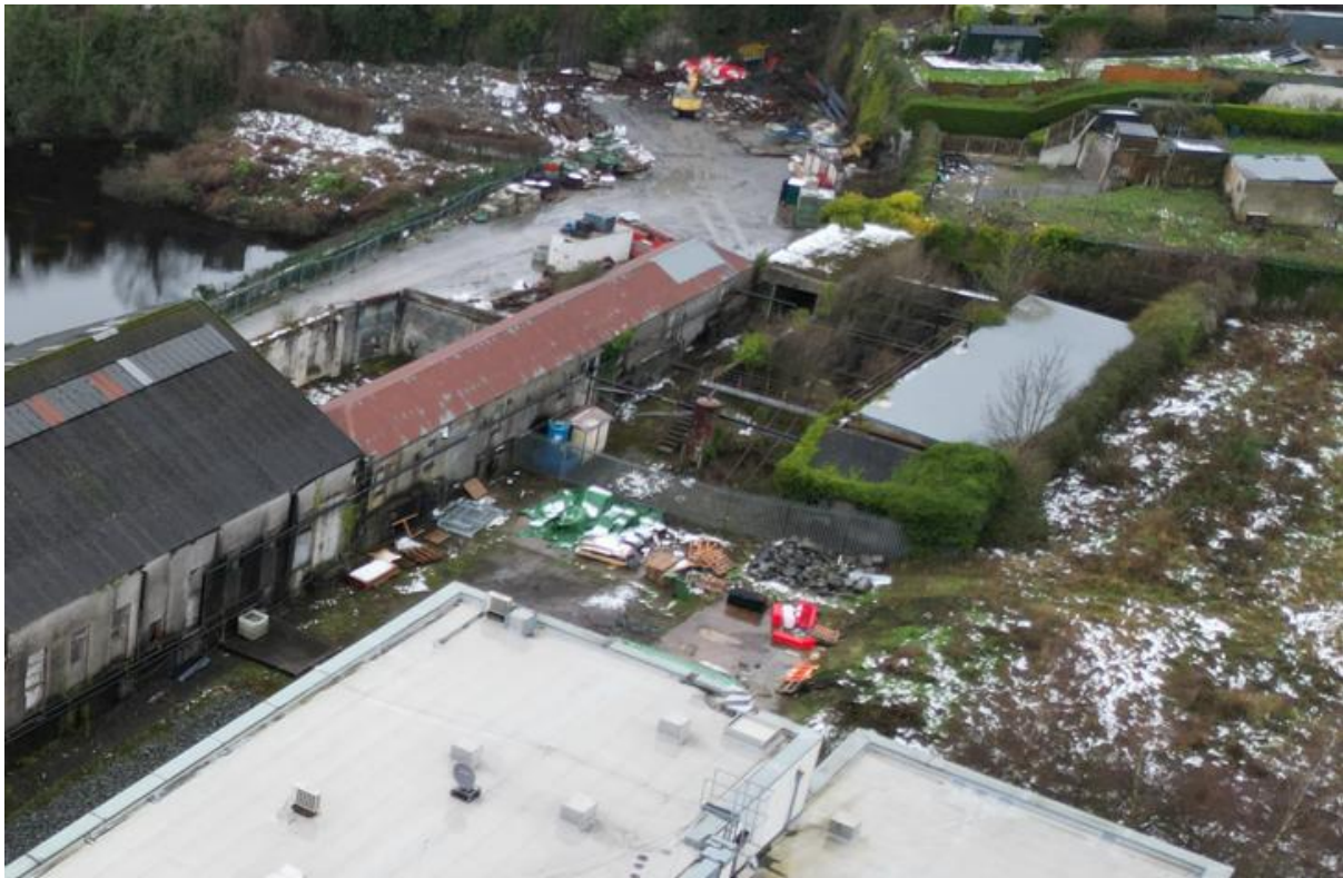
Figure 37 – Aerial of the upper reservoir.
