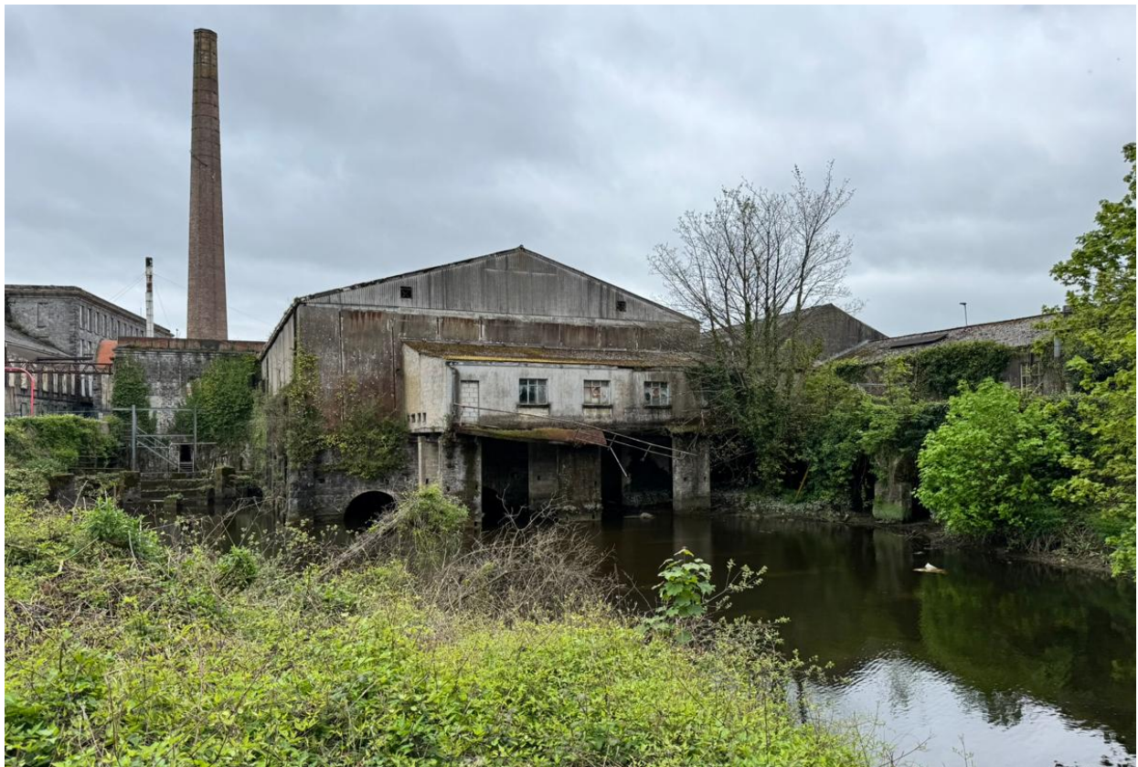
Figure 22 - View across the reservoir to the rear of the infiltration gallery.
