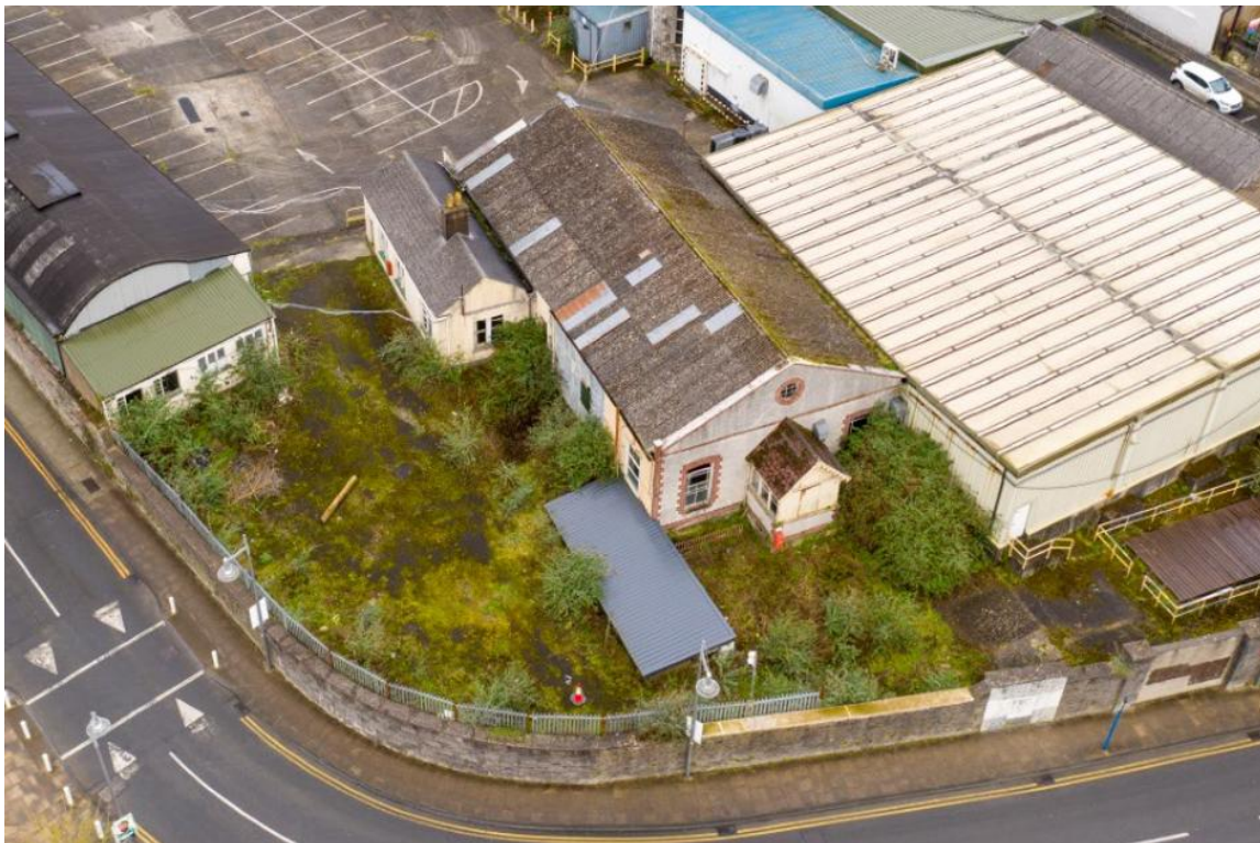
Figure 35 – Aerial of the former Offices and Laboratory.
