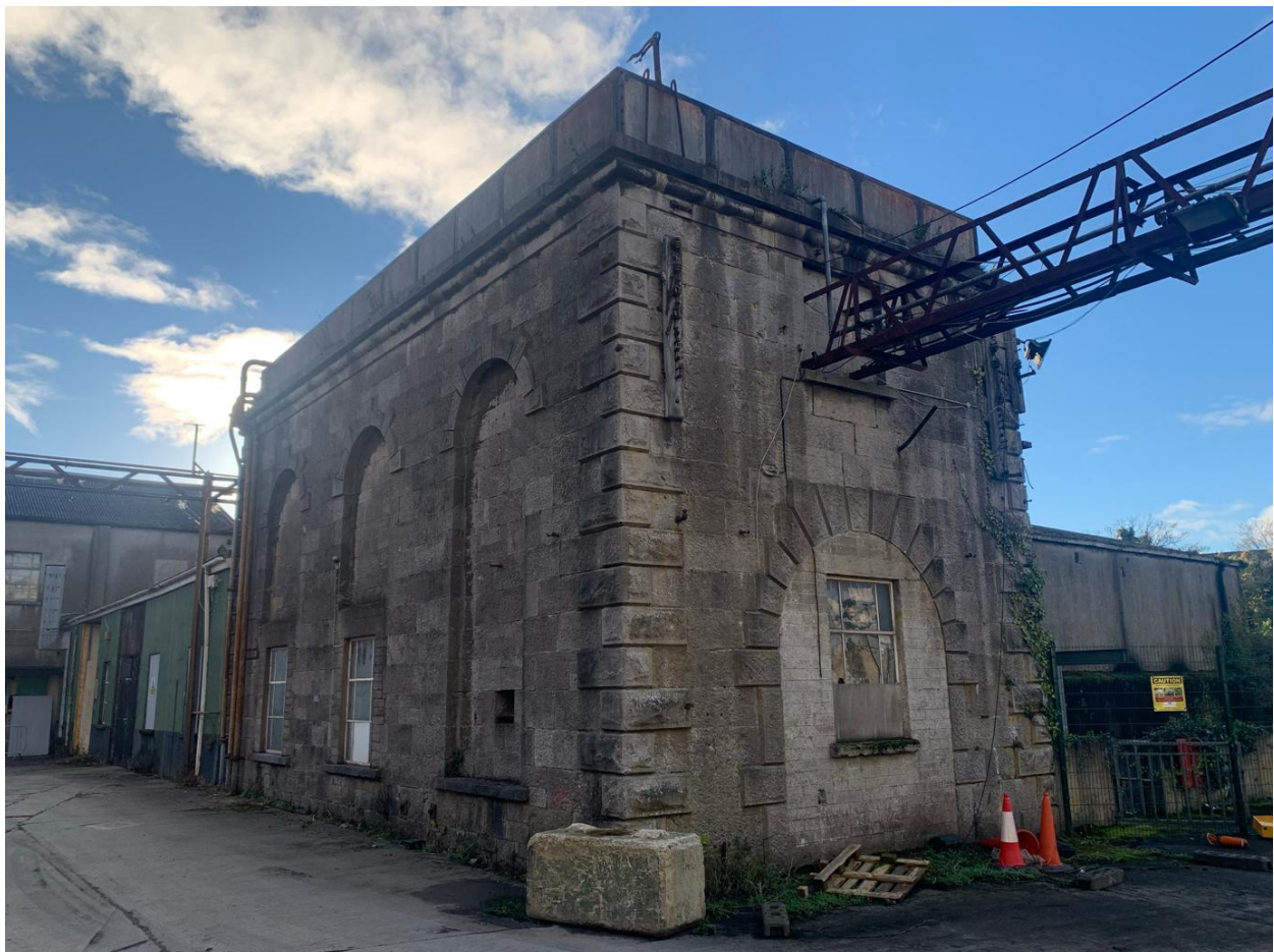
Figure 21 – Watertank building viewed from the north aspect looking south.
