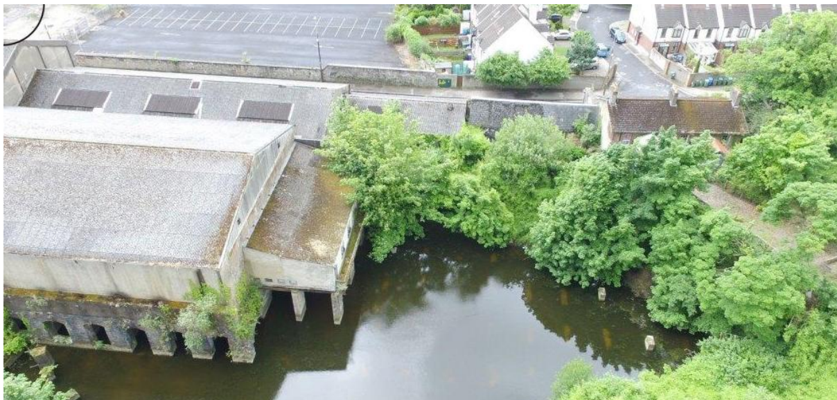
Figure 31 - Aerial view of the Cheese Plant range, between the North Circular Road and the reservoir.
