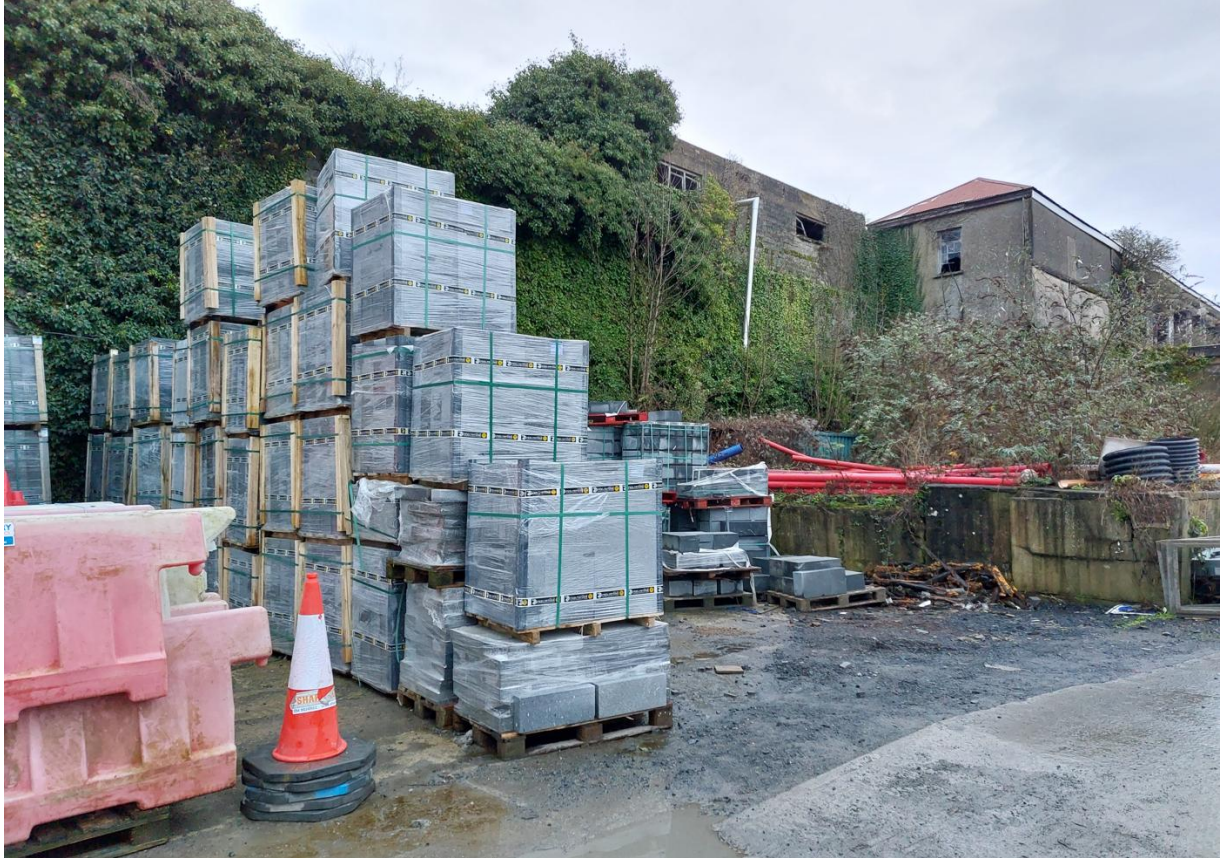
Figure 41 – wall of the quarry toward the former cold store and upper reservoir.
