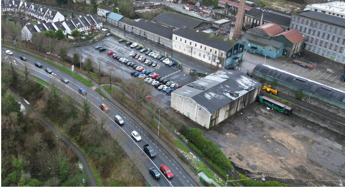
Figure 49 – Aerial of former Shipyard Site.
