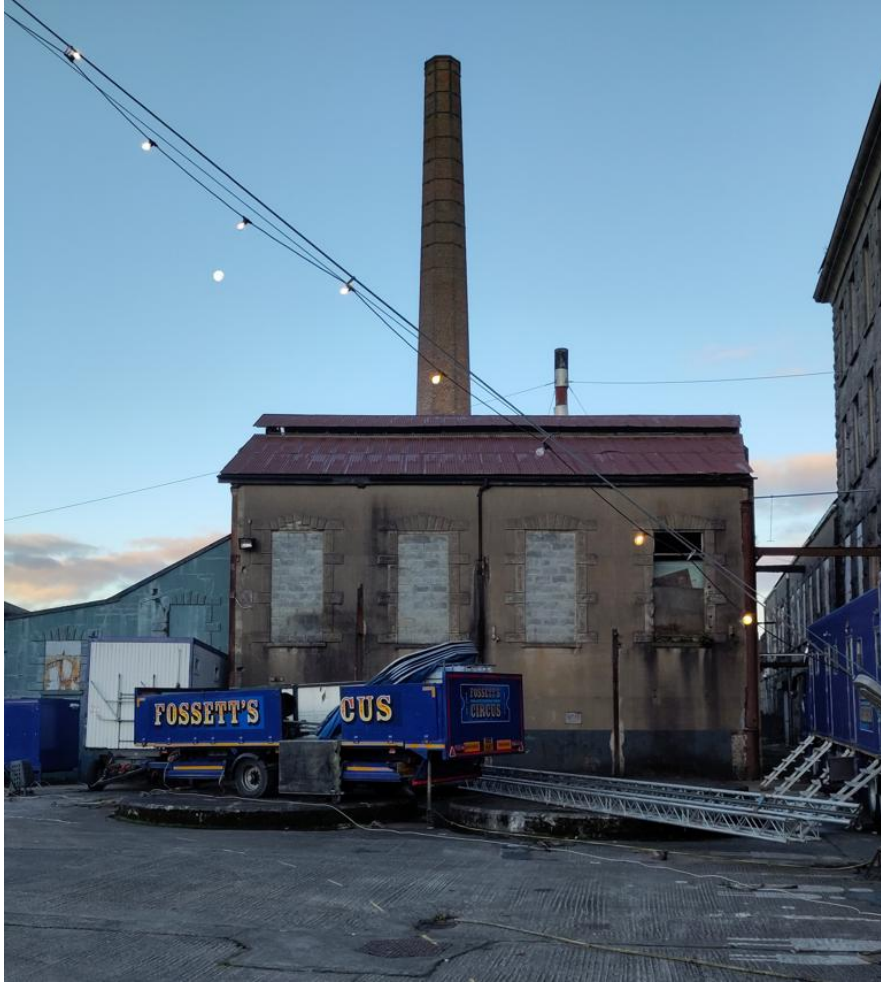
Figure 19 – Front (southeast) aspect of the former boiler house, showing the 1930s extension.
