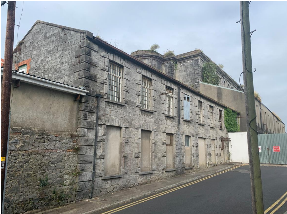
Figure 29 – 1855 Office + Counting House addressing Stonetown Terrace. Original staff entrance 5th bay along.
