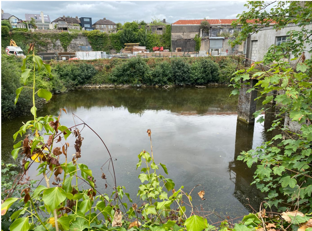
Figure 23 - View across the reservoir from the rear of the Cheese Plant long building, looking north toward the quarry wall.
