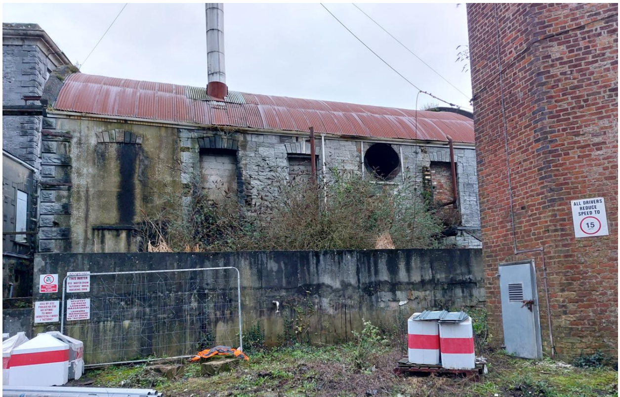
Figure 18 – Rear (northwest) aspect of the former boiler house.
