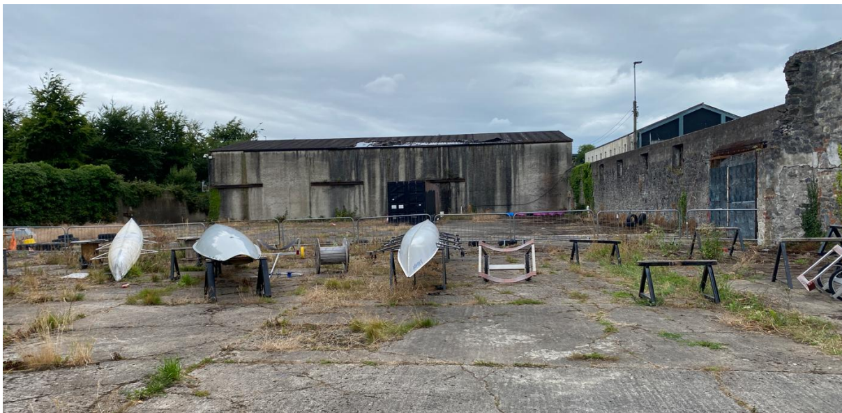
Figure 50 – View from within the former Shipyard site looking toward the warehouse.
