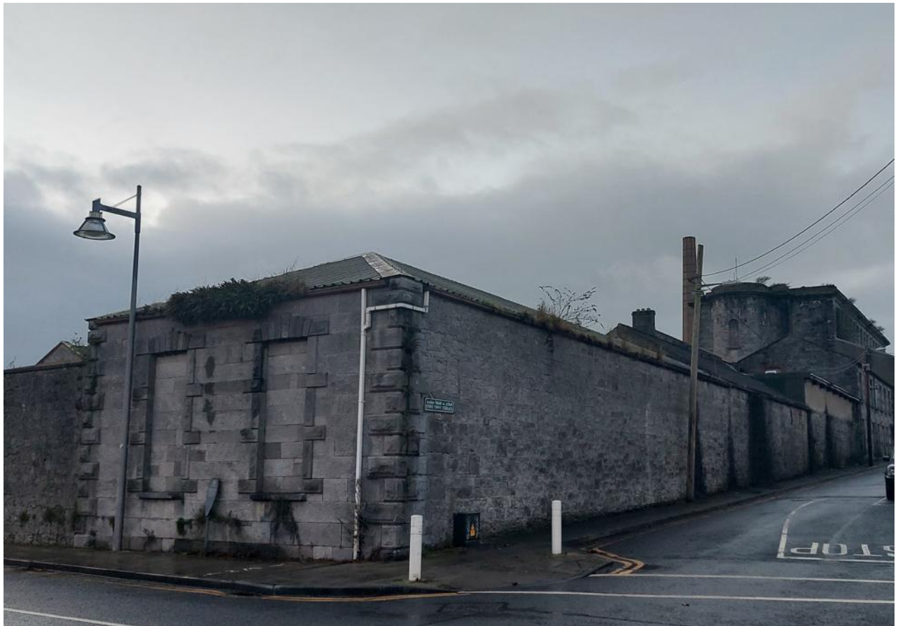
Figure 25 - Former Linen Store, external walls as seen from O’Callaghan Strand.
