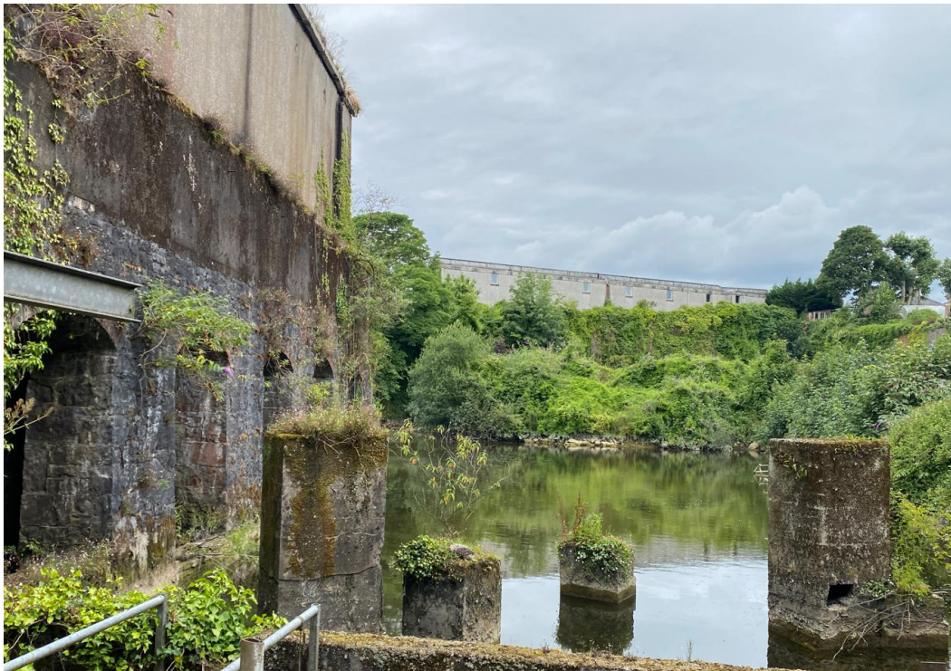
Figure 24 - View across the reservoir from the rear of the water tank, looking west toward the quarry wall and the rear of Former Salesians Secondary School on the higher ground above.
