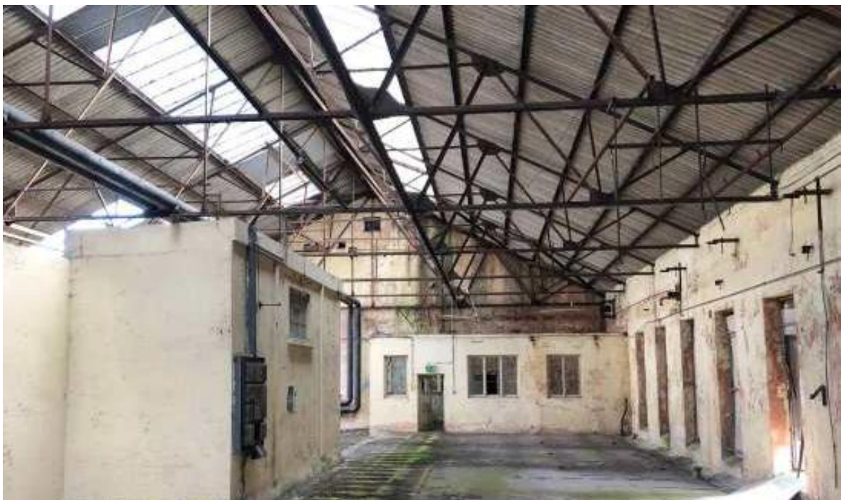
Figure 15 - Interior of the first floor, over the former Weaving Mill.
